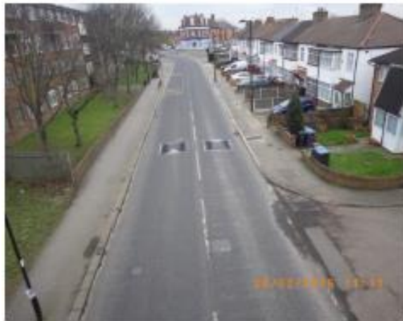
Figure 1 Alma Road before
