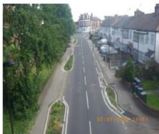
Figure 2 Alma Road after
