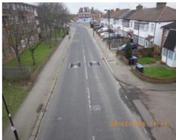
Figure 1 Alma Road before
