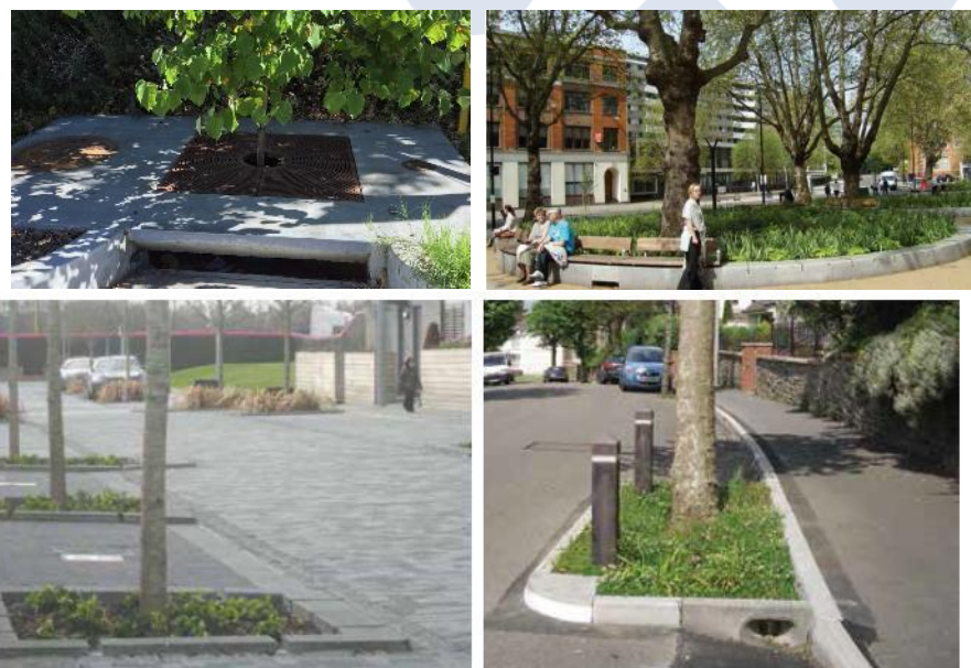
Figure 19.16 Examples of inlets to allow surface water runoff to infiltrate into tree pits (courtesy Anne Jaluzot and Dŵr Cymru Welsh Water)
